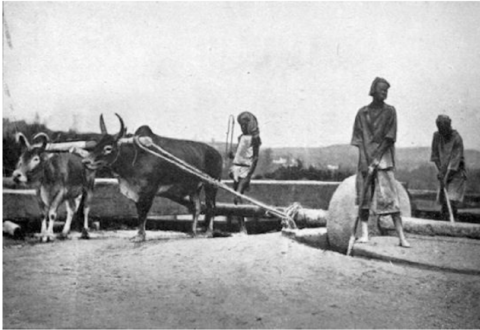
Figure 2 Mortar mill used while building the Government House, Singapore. (Source: McNair and Bayliss, 1899).
