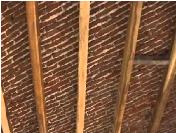
Figure 3 Inside view of Madras-terrace roof. (Source: https://www.pinterest.com.au/pin/36697306-9635001123 ).
