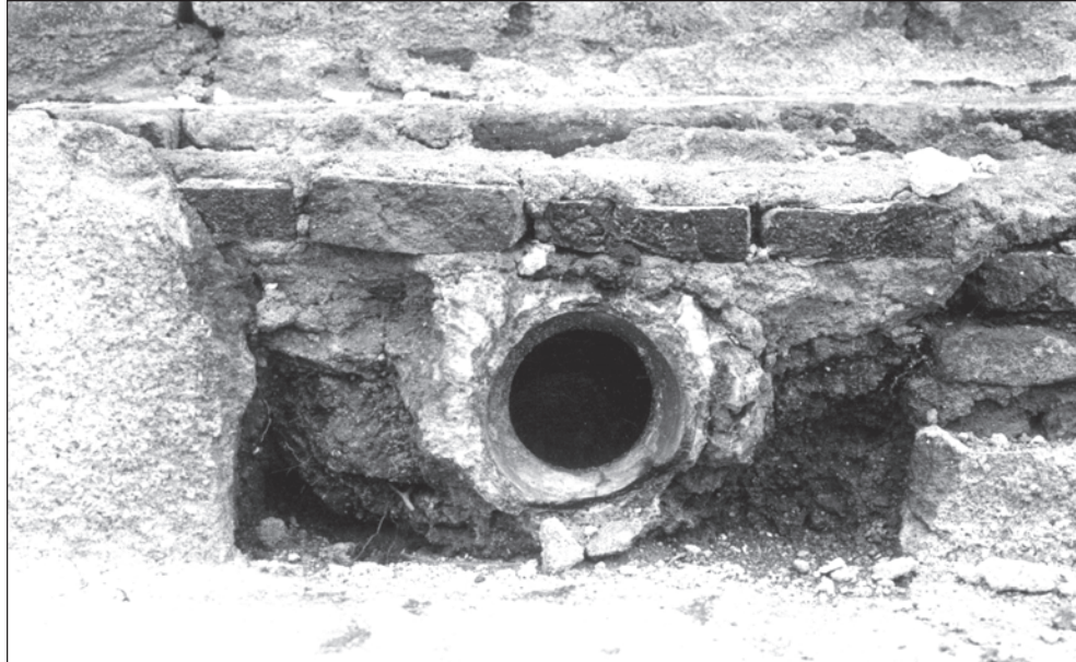
Fig. 4. Kalyanamahal : Earthenware pipe (south side), opening
