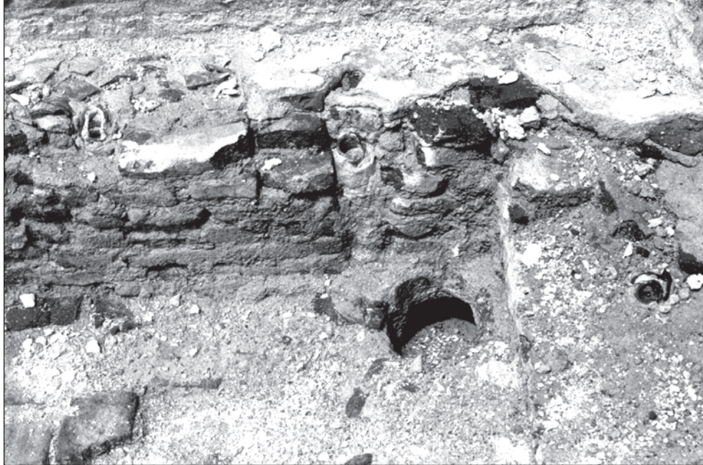
Fig. 2. Kalyanamahal : Earthenware pipe (north side), heavy brickwork, hole for vertical pipe
